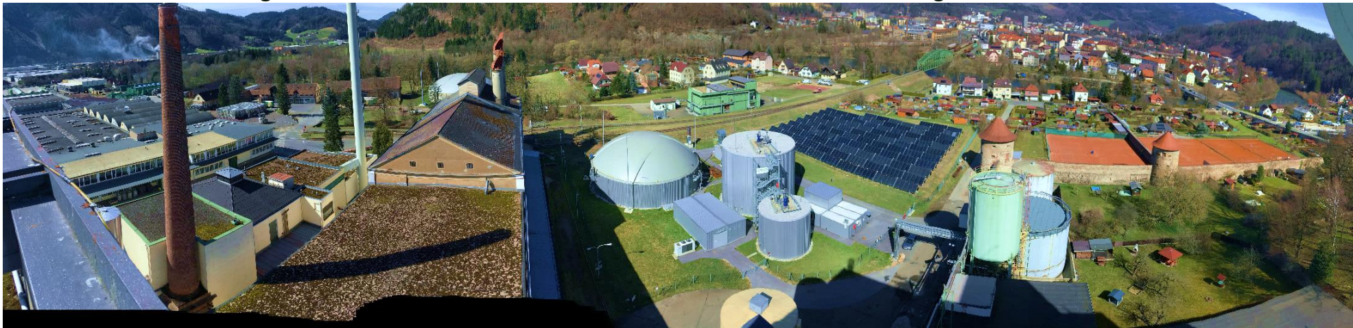
Goess brewery sustainable energy supply surrounding
